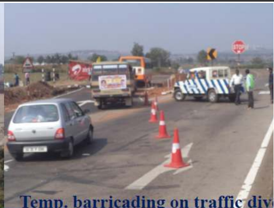
Barricading on traffic diversion
